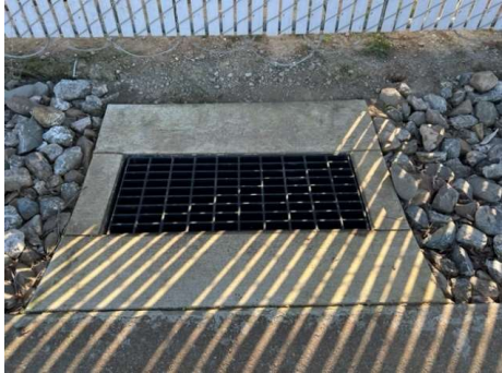
Drop Inlet / North Trench
