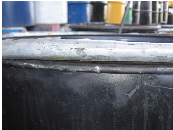
Drum ring is not properly secured. Notice drip lines on side of drum.
