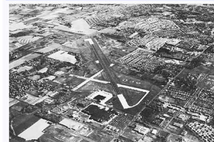
Aerial view of the NADC in the early 1970s
