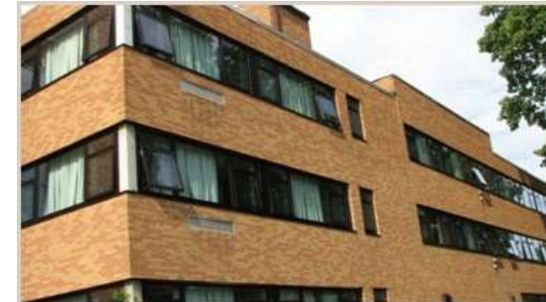
Since the project's start in 2011, new windows have been installed in Dunbar, Prentice, Verder, Lake, and Olson Halls.
