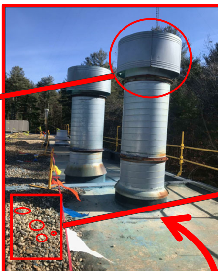
Roof Ballast and Roof Stack
