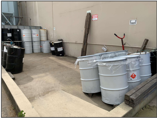
Secondary Containment / Dikes / Berms
