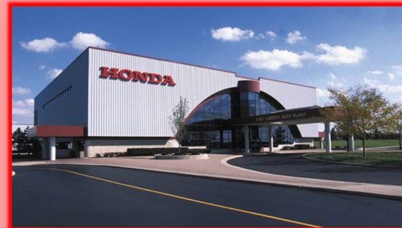
1989 East Liberty Plant
