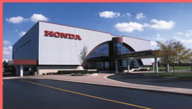
1989 East Liberty Plant
