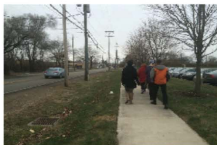
Improved sidewalks on Harmon Ave
